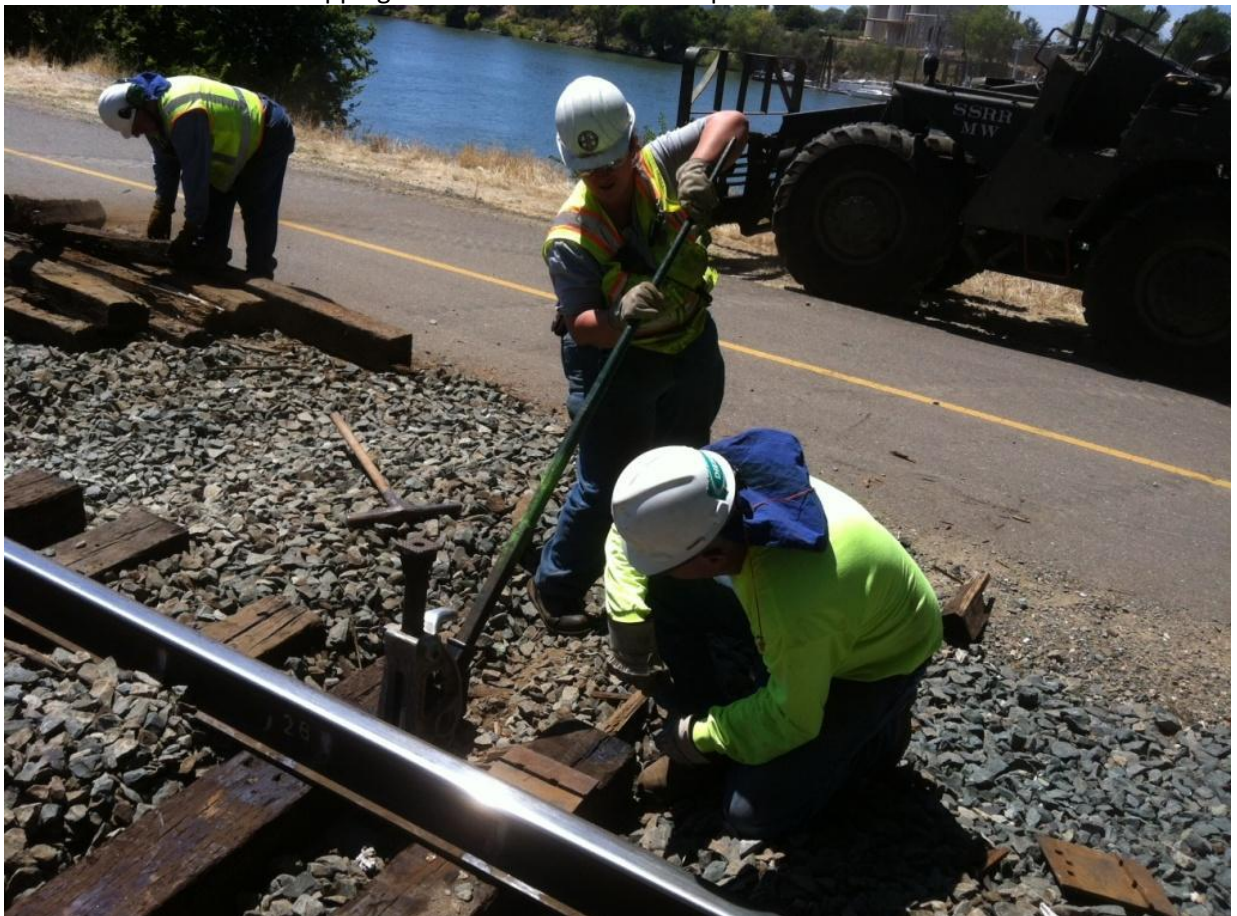
Heather and Dave use a track jack to lift the rail to insert a tie plate.
