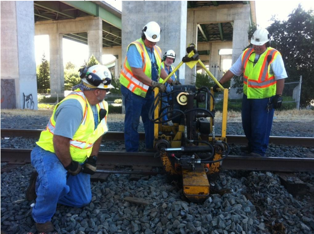
Mike F., Chris, Frank, and Harry extract a tie with the section-gang machine.
