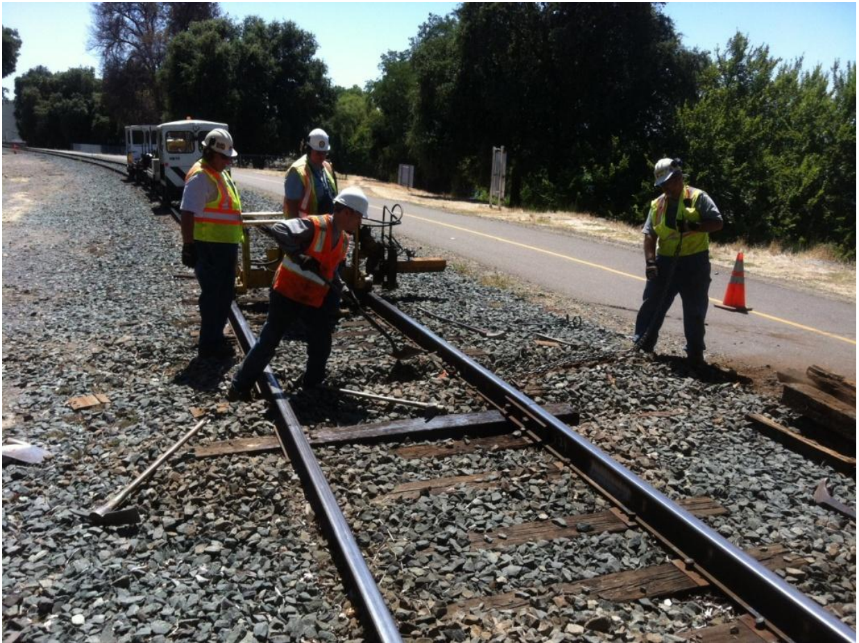
Garrick shovels ballast to deepen the crib for the new tie.
