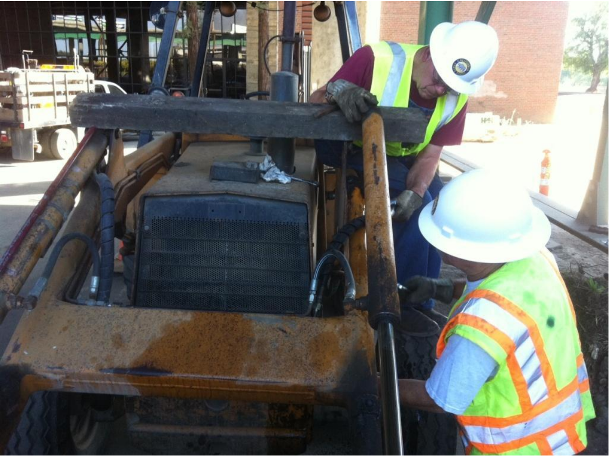
Cliff and Mike take apart the hydraulic cylinder on the back-hoe to repair the blown hose.
