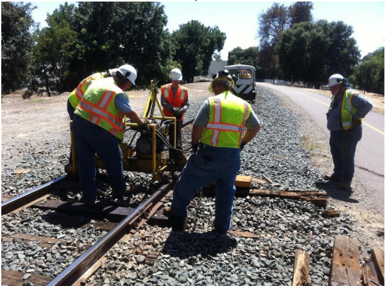
Now the new (well, "newer") tie gets inserted.
