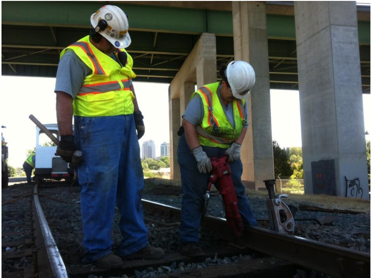
Mike sets the spikes while Heather uses the pneumatic spiker to drive them in.
