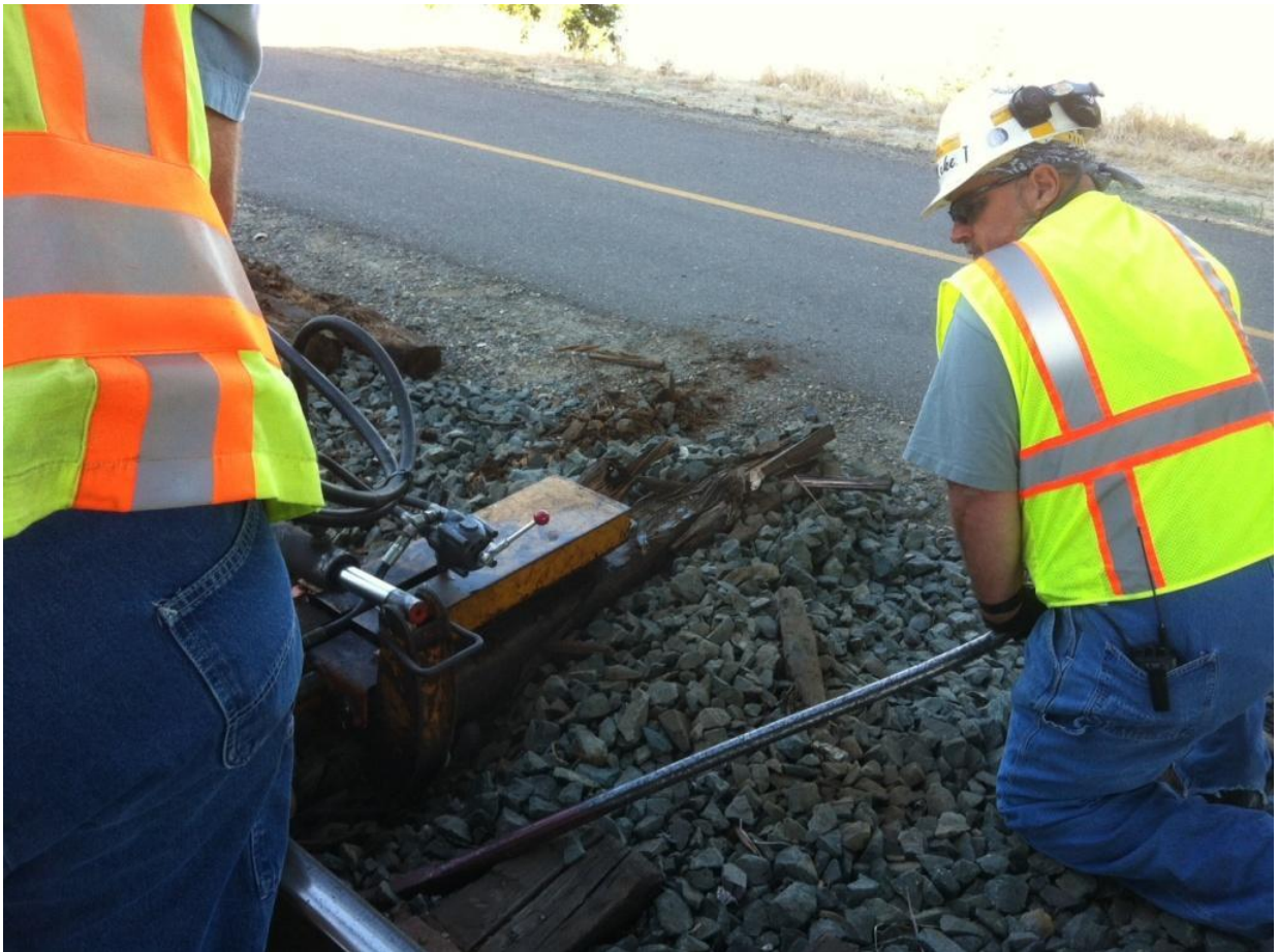
Mike F. uses the nipping bar to lift the rail to relieve pressure as the bad tie is extracted.
